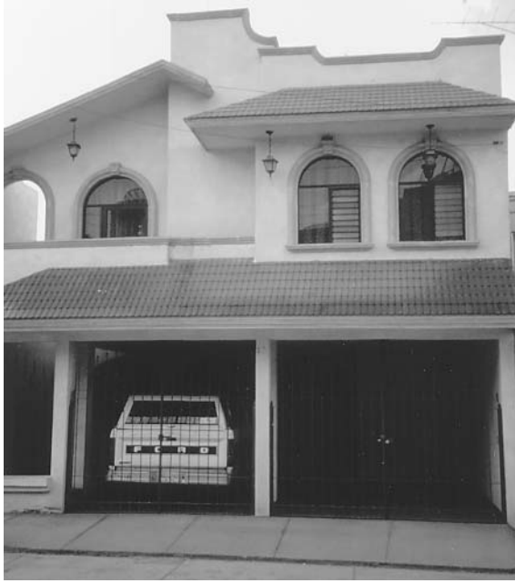
Photograph 2.6. New House. Newer homes reflect new needs, such as a garage for cars purchased through hard labor in the United States. The home pictured here integrates some traditional Mexican design elements (stucco, sandstone trim on the windows and along the roof, a tile roof, and the wrought-iron-and-glass decorative lamps), but also provides room for a two-car garage. The two-story design separates living areas into public and private in a way that is quite distinct from older homes.
